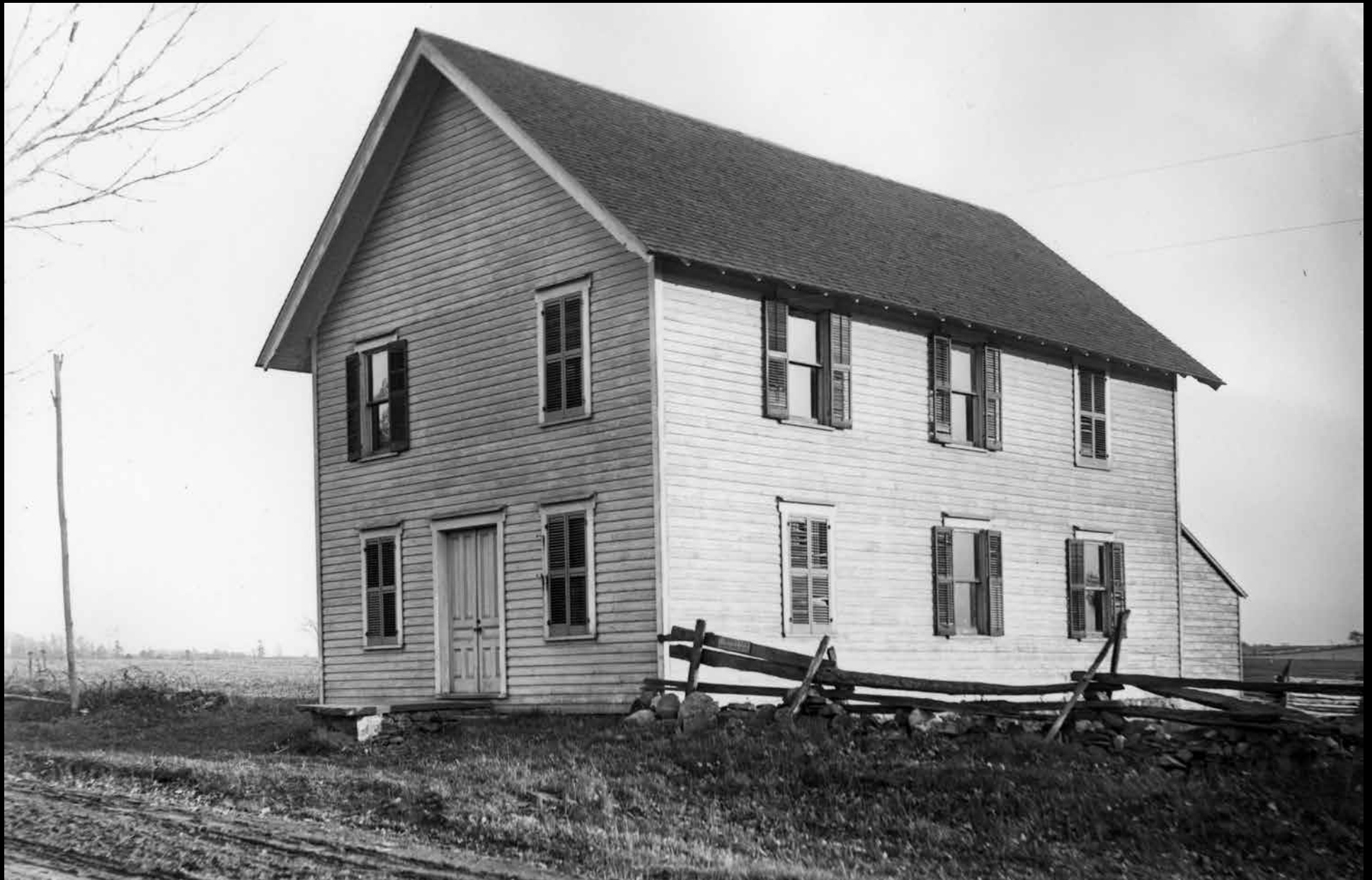
East Lansing Grange Hall, 1907
