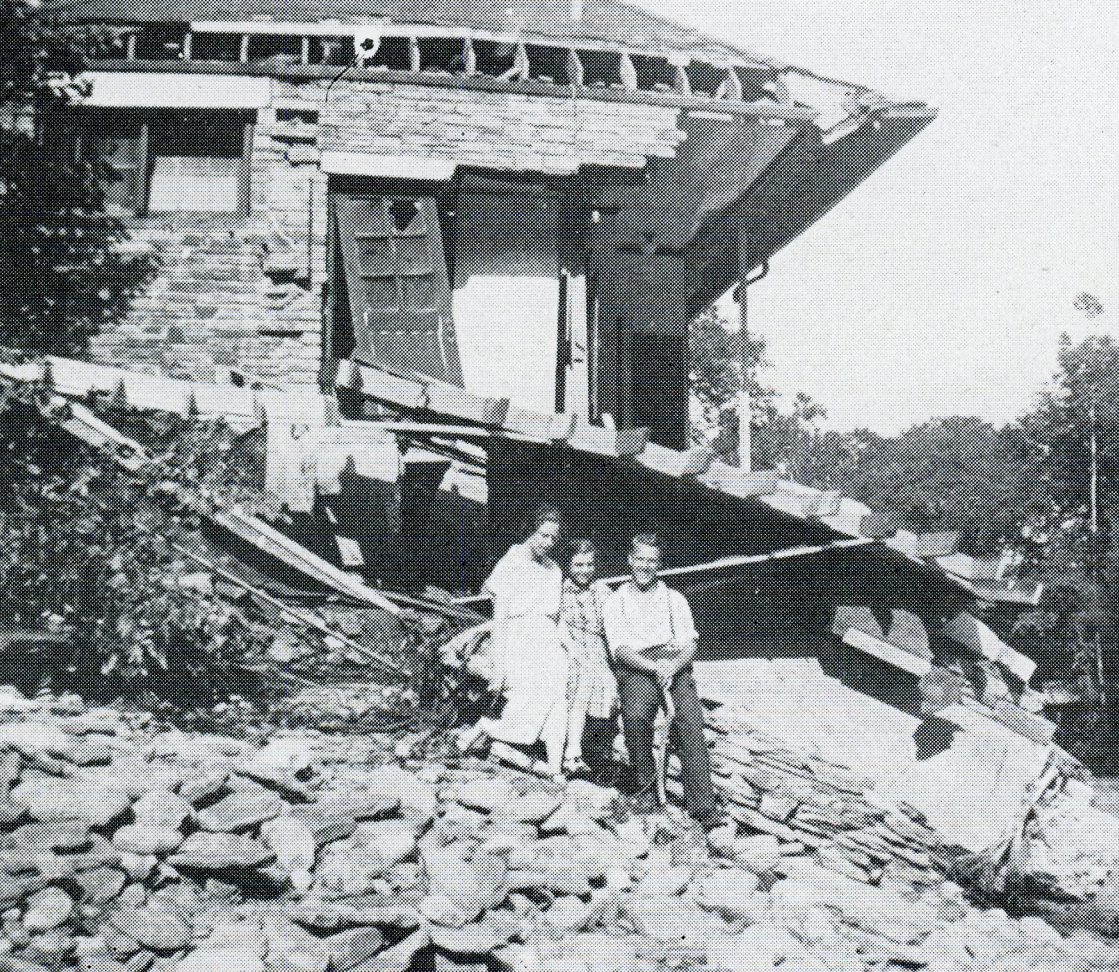
Damaged Bathhouse, Enfield Glen near Ithaca
